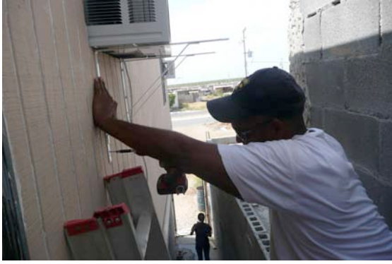
Richard installs air conditioners in classrooms.
