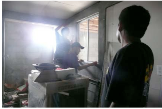
Angel Balderas checks new windows.
